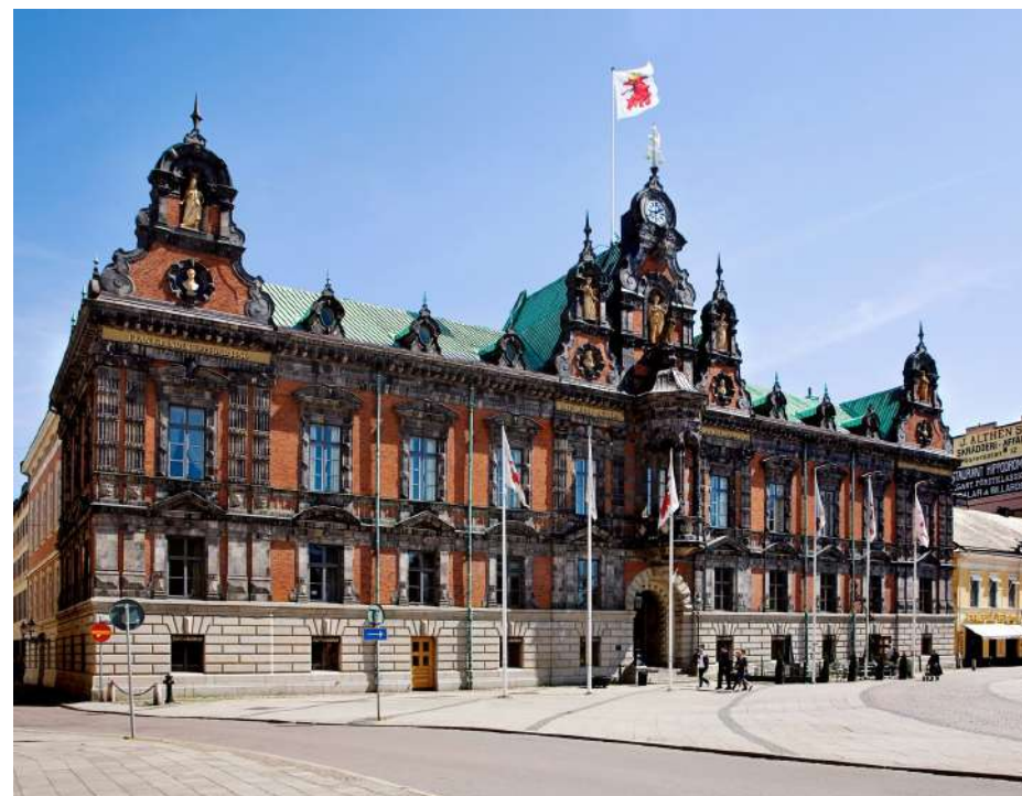
Malmö City Hall, Rådhuset. Photo by Bojana Lukac
